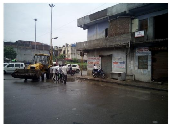
08-FOOTPATH PEDESTRAIN FACILITY.jpg
