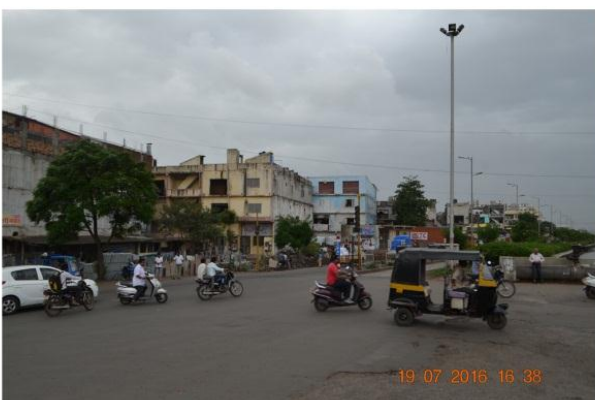
07-CONDITION OF ROAD.JPG
