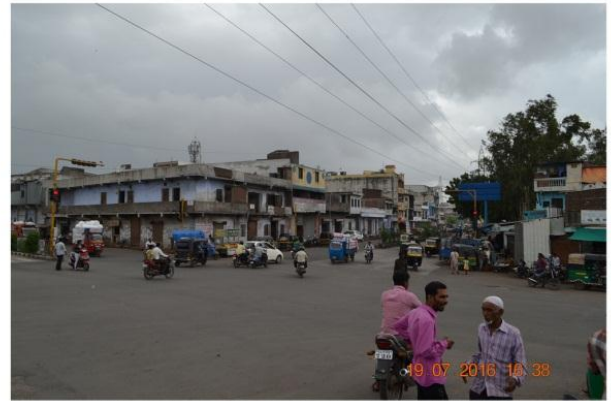
02-CONDITION OF CARRIAGEWAY.JPG
