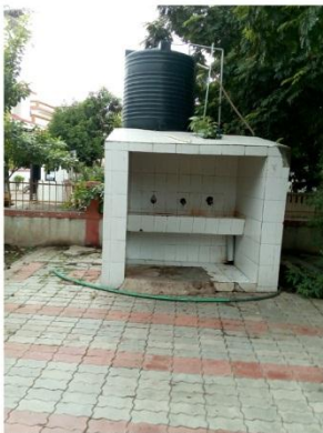
19-CONDITION OF DRINKING WATER FACILITY.jpg
