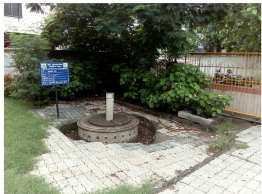
16-EXISTING RAIN WATER HARVESTING CONDITION.jpg
