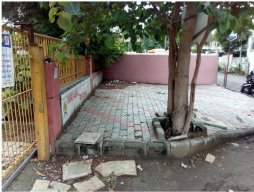
17-PARKING AT SECONDARY ENTRANCE GATE.jpg
