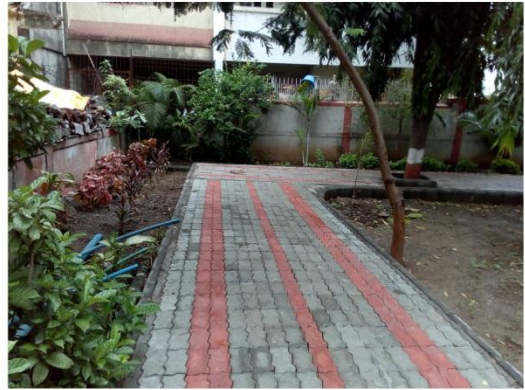
10-CONDITION OF BOUNDARY WALL.jpg
