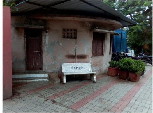
02-EXISTING CARE TAKER ROOM.jpg
